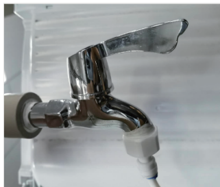
Step 7) Screw the water pipe into the faucet (can sealed with tape).
